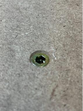
2. **Note:** The holes are countersunk such that the threaded insert will sit about 1mm from the plane of the MDF.
